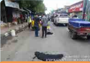
Januari | January Kegiatan Perbaikan Jalan (patching) Road Repair Work (Patching)
