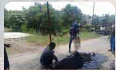
Desember | December CSR Kegiatan Perbaikan Jalan Lingkungan di Desa Mranak CSR Community Road Repair Project in Mranak Village
